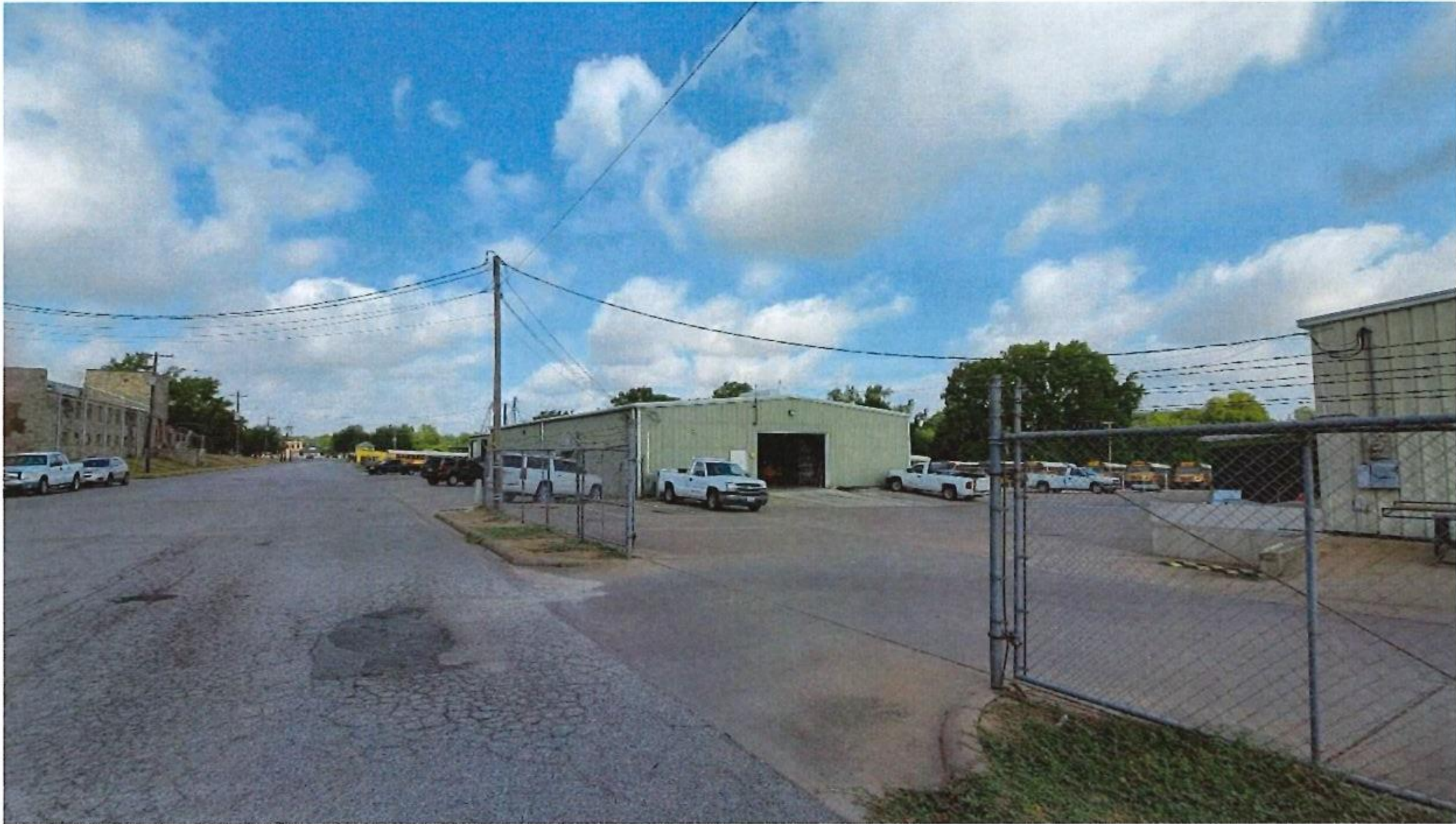
BISD Transportation Depot & Rock Gym
